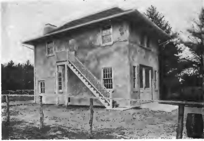
EXTERIOR OF THE MORRIS GARAGE AT WESTCHESTER, N. Y.
